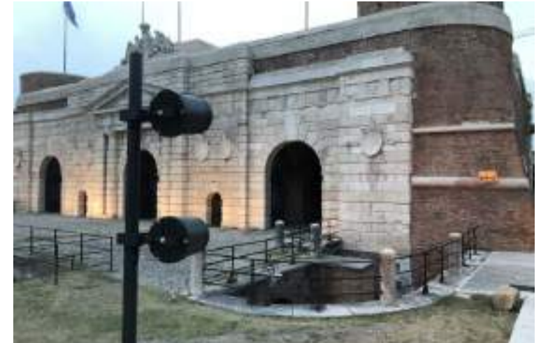
retrofit targeted interventions on existing installations, guaranteed continuity
